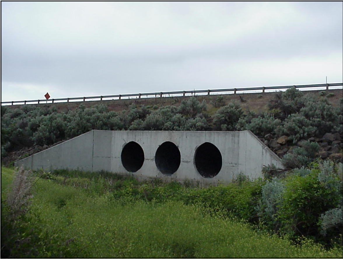
Upstream entrance of 3-culvert conveyance with concrete headwall
