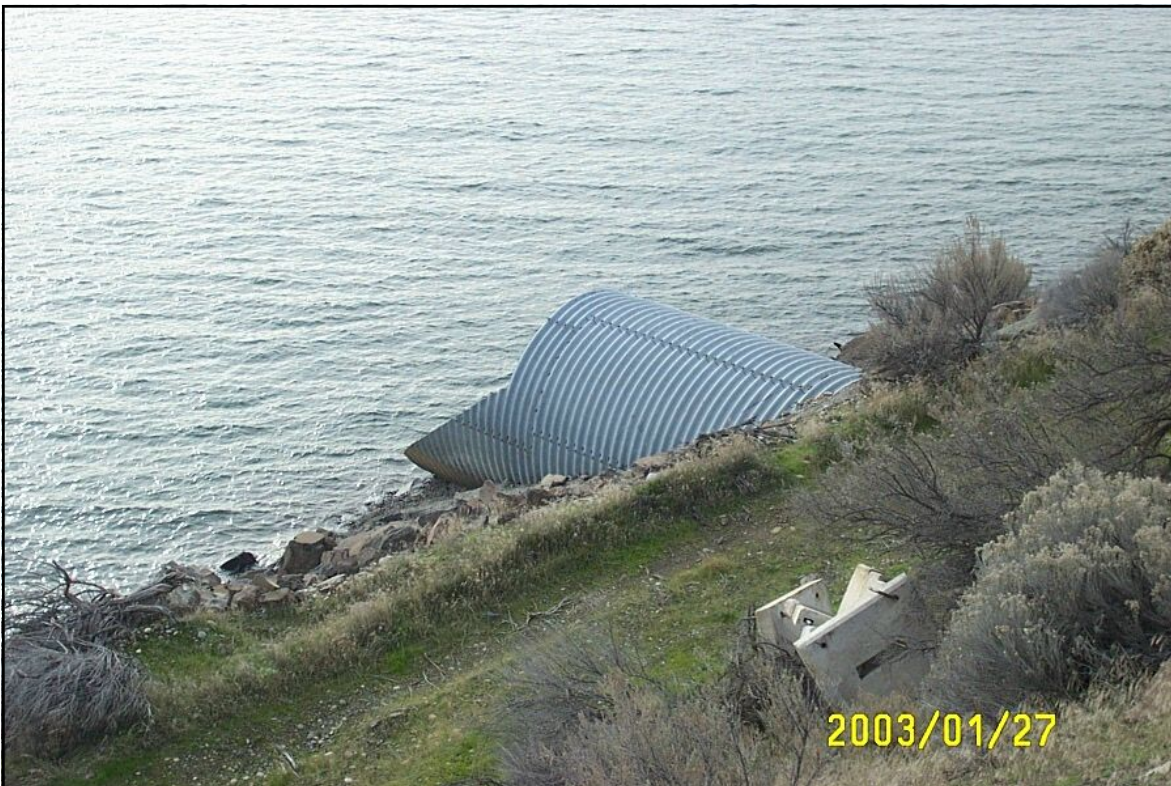
West culvert discharge
