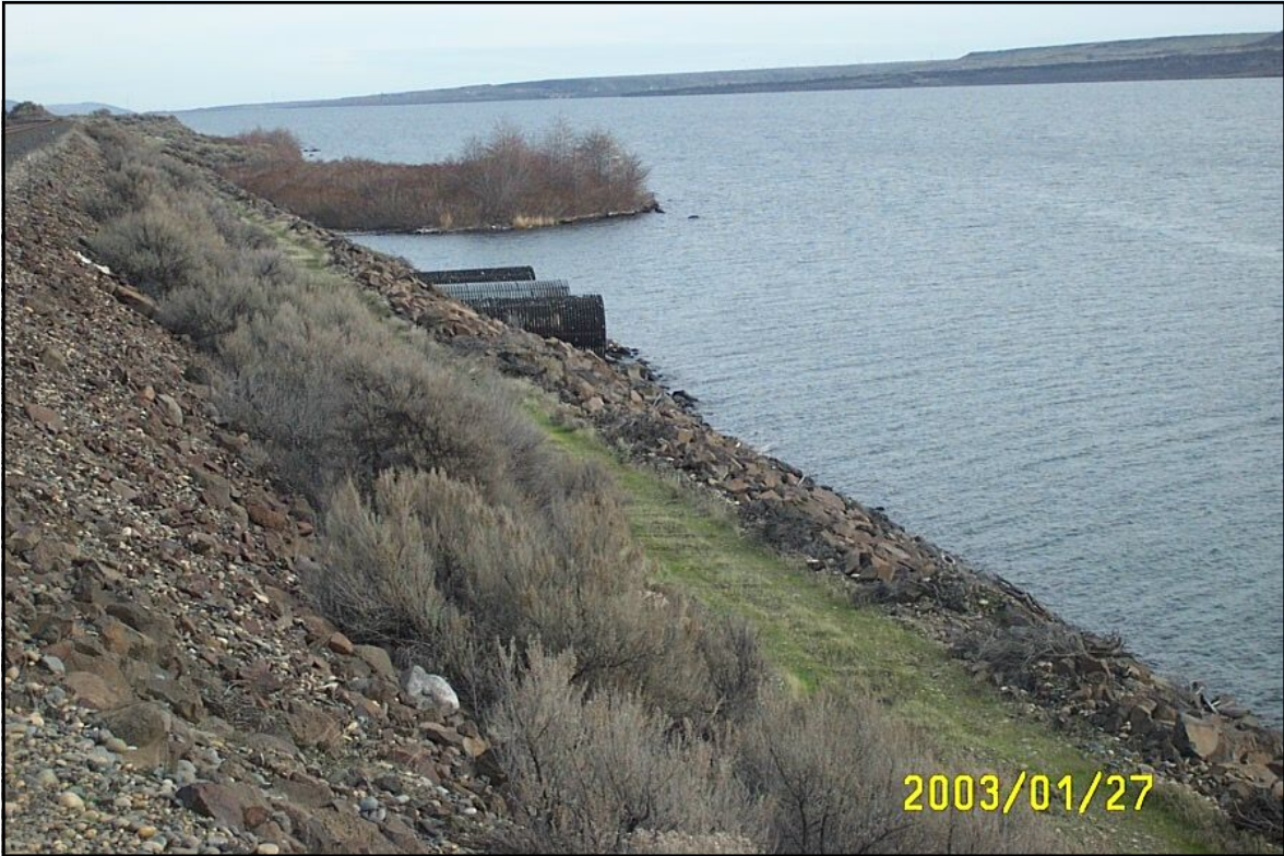
Downstream discharge of 3-culvert conveyance into Columbia River
